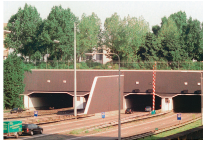
FIGURE 7 The Drecht Tunnel under the Oude Maas River in Dordrecht blocks satellite signal reception over a distance of more than 550 meters.
