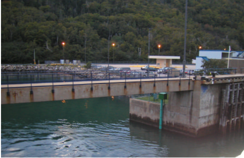
Figure 13 – Tide gauge station in Digby
