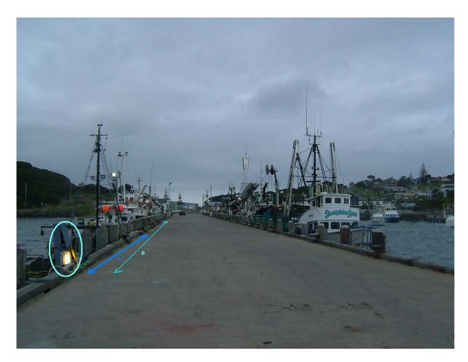
Figure 3.6 Wharf with ships at berthed, showing a power outlet. The power outlet in this wharf can be suitable for ships berthed at a distance "a" from it. But a ship berthed at a distance "b" from the power outlet must make sure that her power cable length is long enough to reach the power outlet
