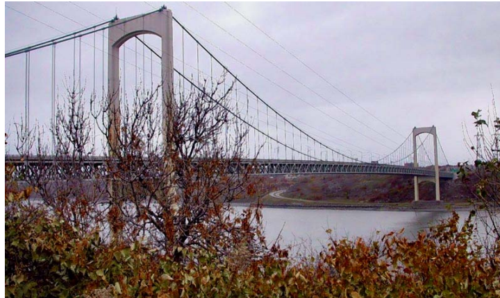
Figure 1. Pierre-Laporte Bridge, near Quebec City, Canada ( http://www.trekearth.com/gallery/North_America/Canada/photo30284.htm )
