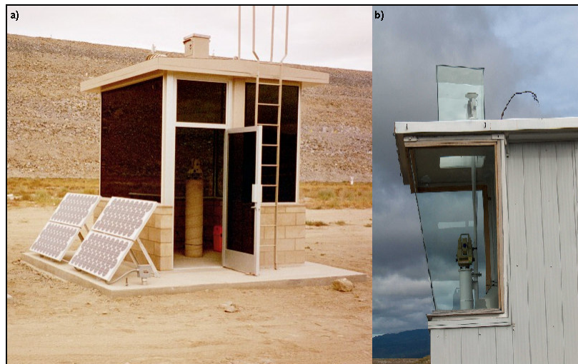
Figure 2: a) RTS shelter with solar power panels, b) Typical RTS/GPS ALERT shelter
